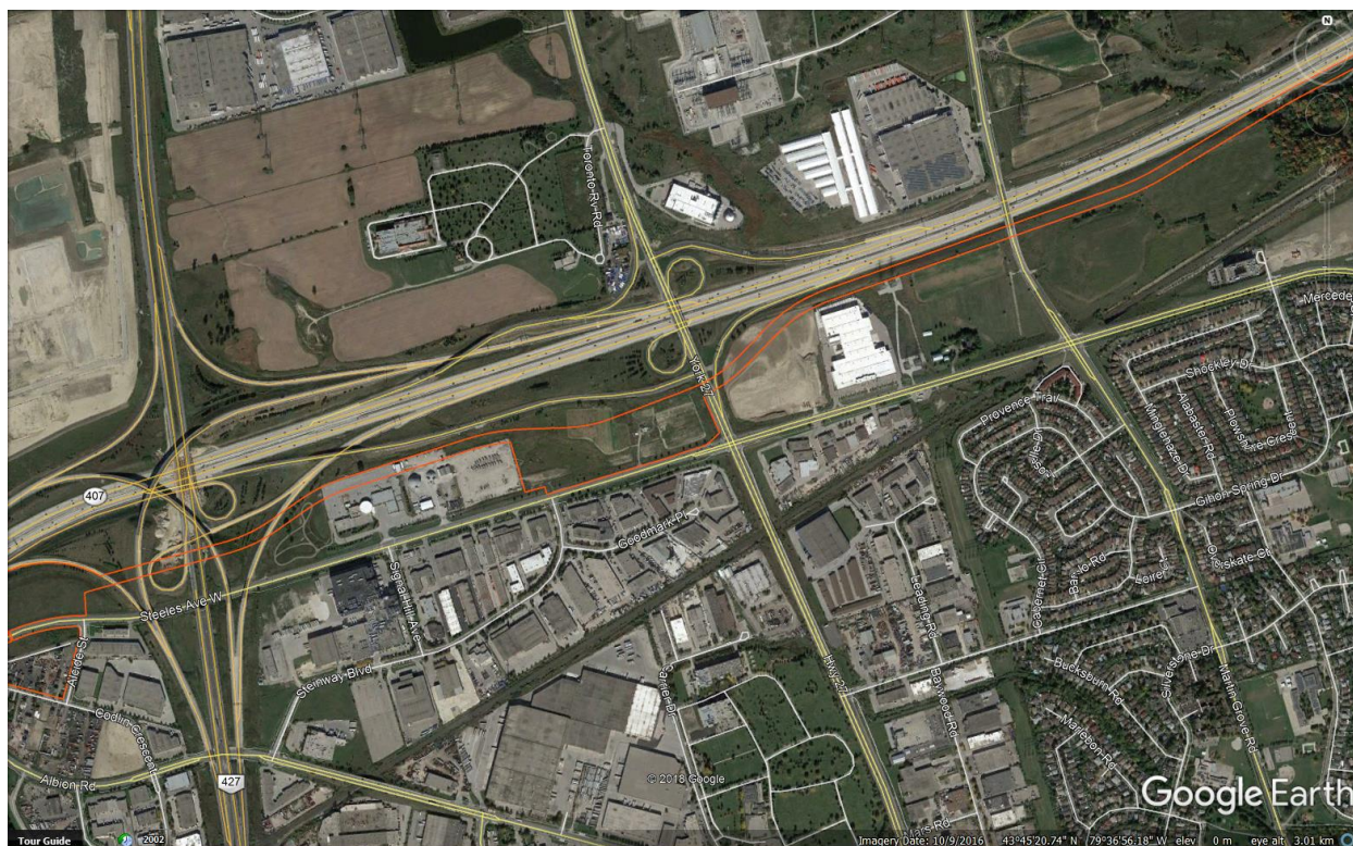
FIGURE 15. SEGMENT F AIR PHOTO AND 407 TRANSITWAY FOOTPRINT
